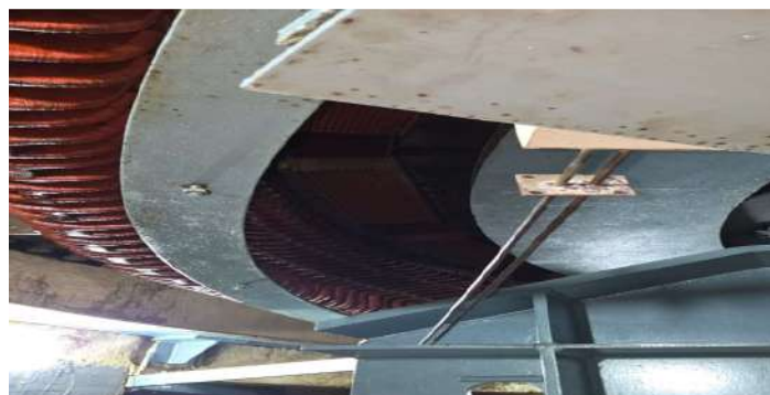
Heating arrangement of Top Bracket
