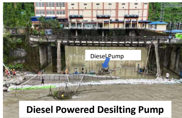
Desilting work view from Tail pool side
