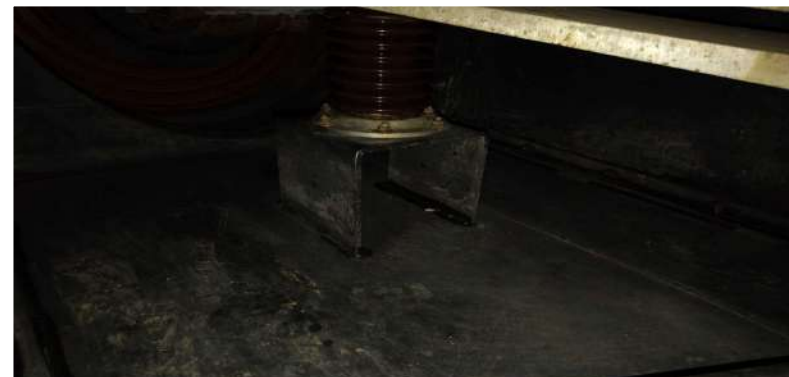
Cleaning of Line Side Busduct
