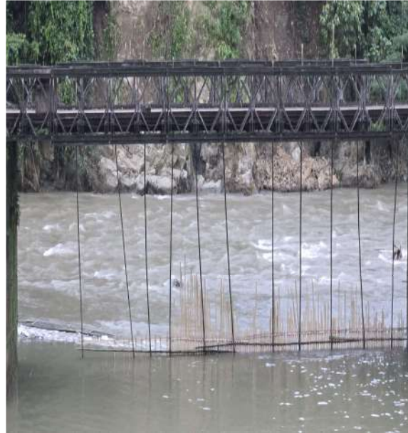
Photo of Temporary Barrier
