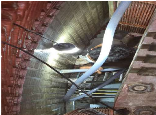
Cleaning of Stator
