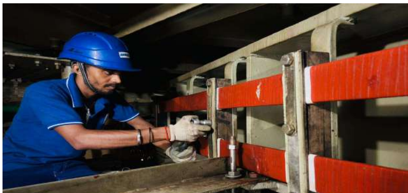
Cleaning of DC Lead
