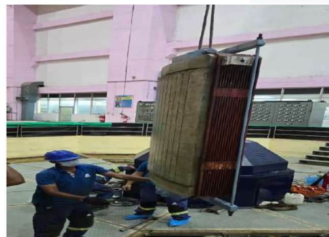
Removal of Rotor Pole
