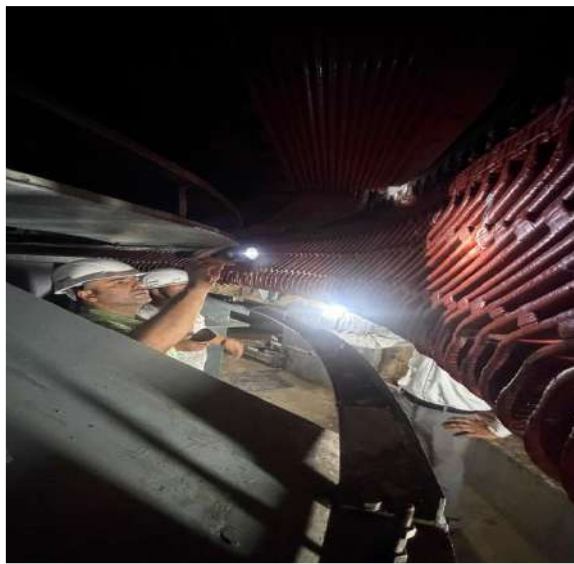
Stator Overhang Portion
