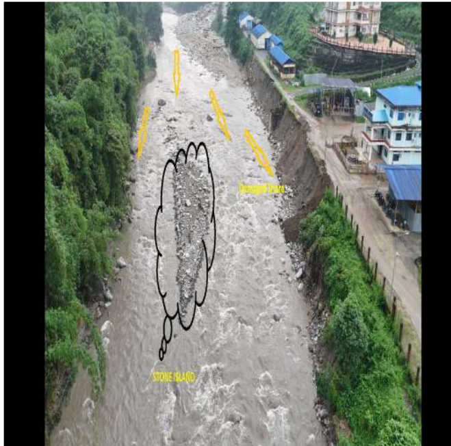
Dikrong River and Damaged Protection wall
