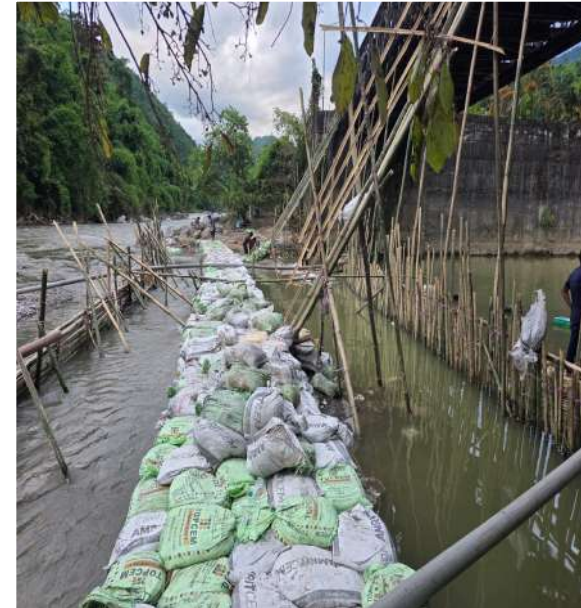
Photo of Temporary Barrier
