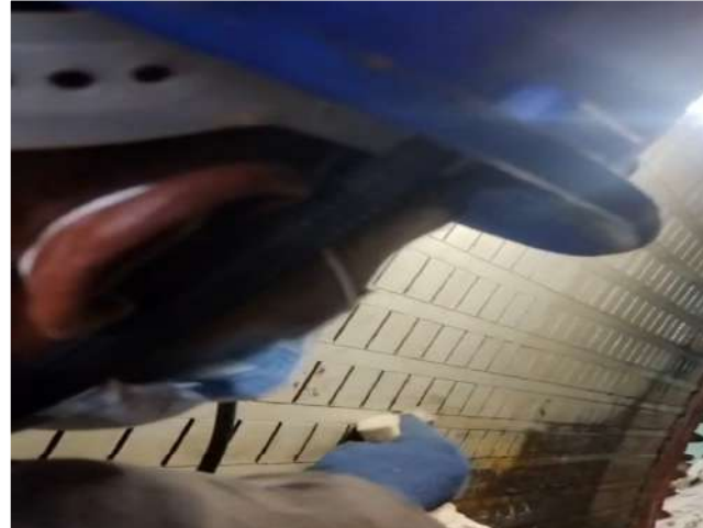
Cleaning of Stator
