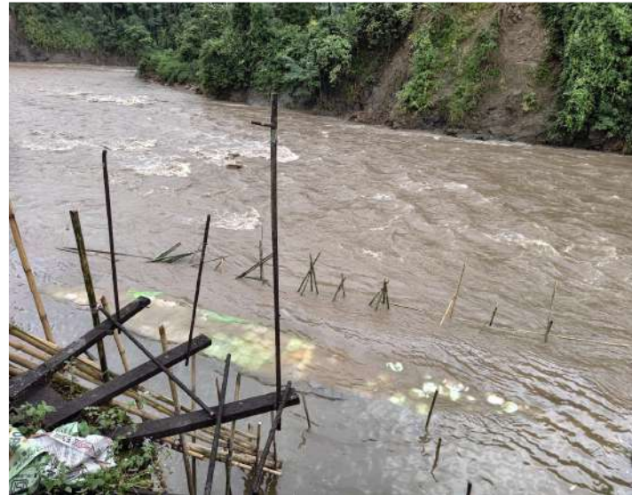
Temporary Barrier Submerged Due HFL in Dikrong River on 12.07.2026
