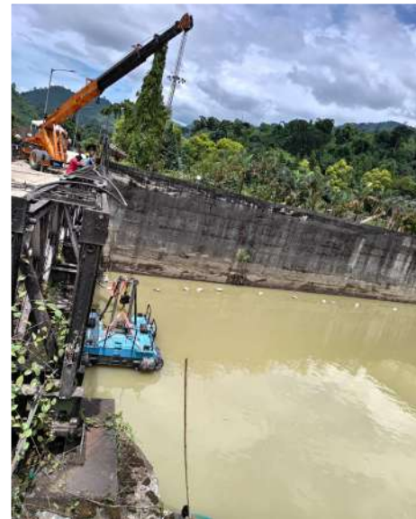
Automatic Dredging/desilting 60 HP Electric Pump
