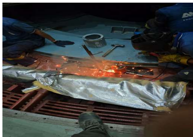
Arrangement of removing of Rotor Pole
