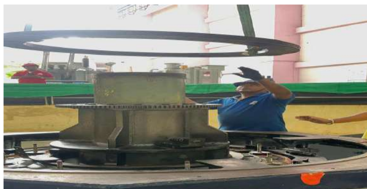
Removal of Slip Ring
