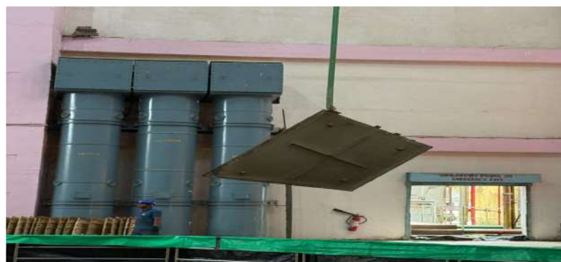
Removal of Chequered Plates
