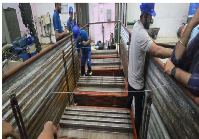
Heating arrangement of Pole
