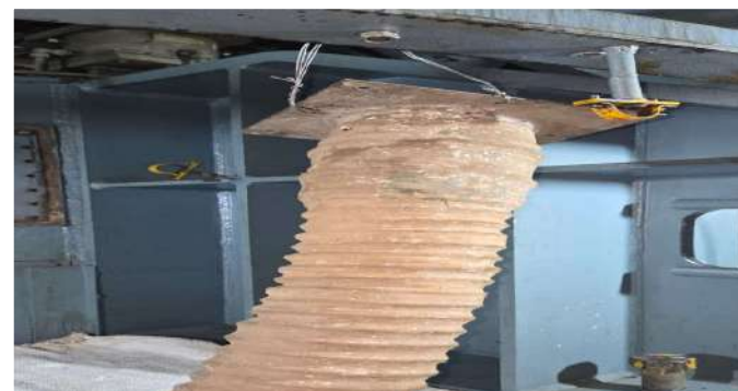
Heating arrangement of Lower Bottom Bracket
