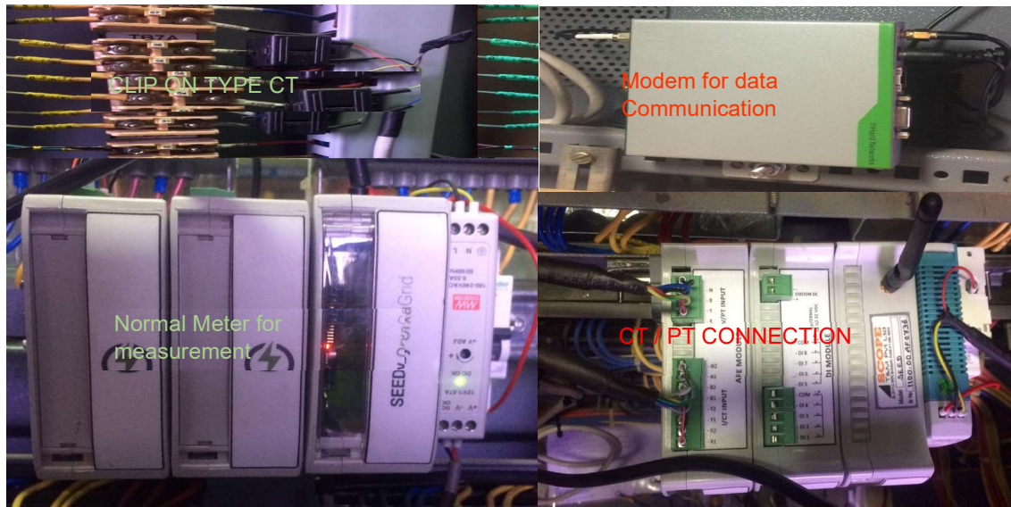
Fig 2.3: Site Installation Photos of Pilot Scheme 1 of GETCO
