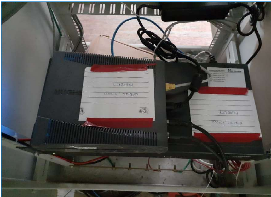
Figure 6: VSAT IDU and Terminal Server at Killing substation under Pilot Project
