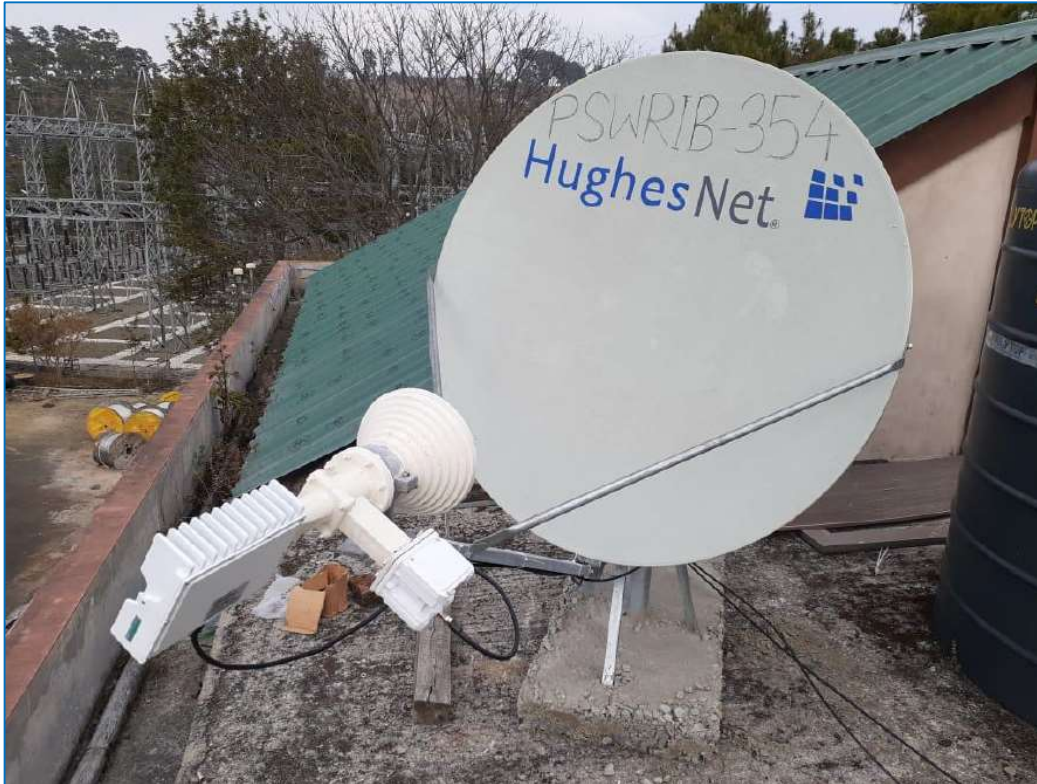
Figure 5: VSAT antenna installed at Meghalaya-SLDC (at NEHU) substation under Pilot Project
