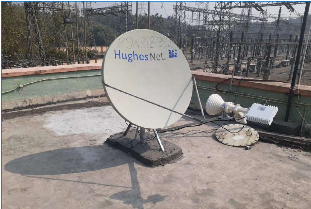
Figure 4: VSAT antenna installed at Killing substation under Pilot Project
