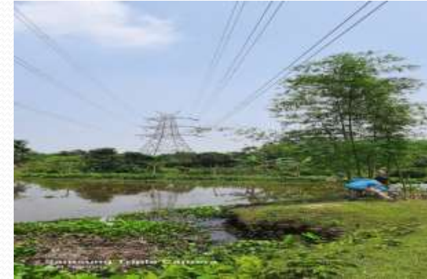
Vegetation infringement under the line corridor
