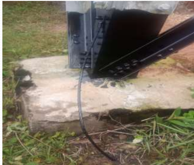
Application of (Anti-Corrosive) to avoid further rusting of CP earthing.
