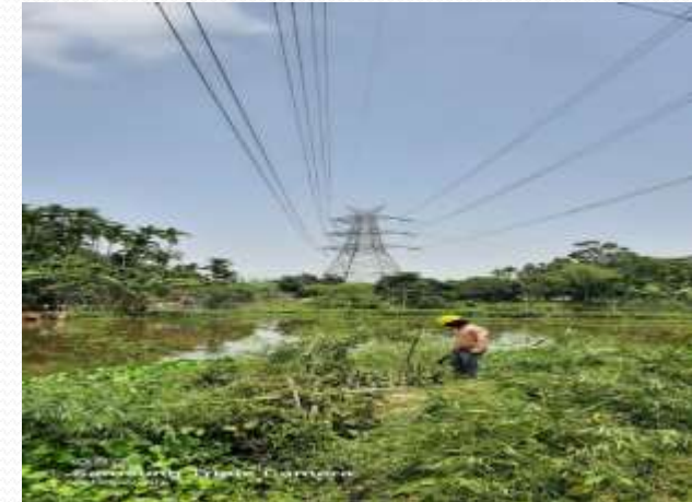
After clearing the vegetation infringement
