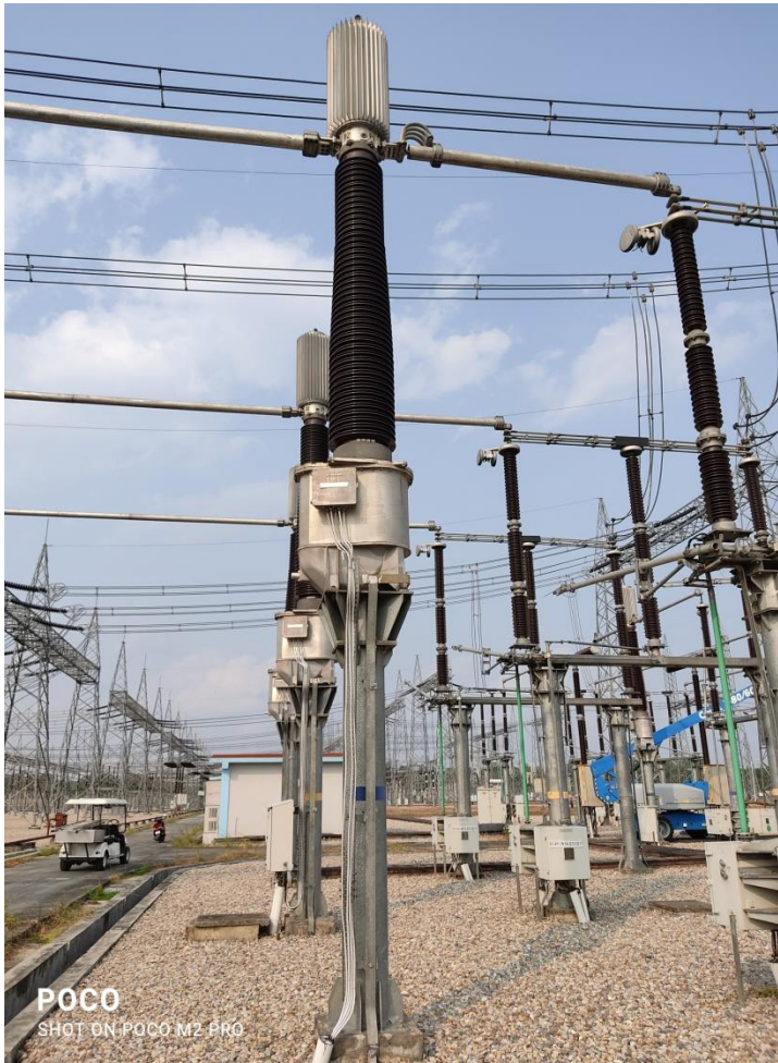
Installed 400 kV CT
