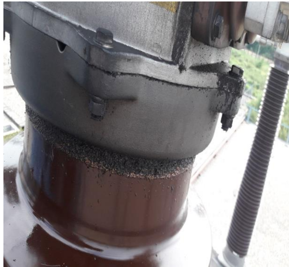
CT oil leakage pics detected by visual inspection
