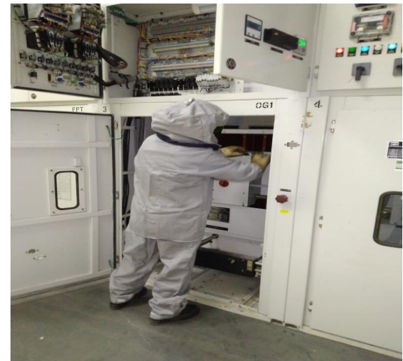
Use of Arc Flash suit at HVDC BNC
