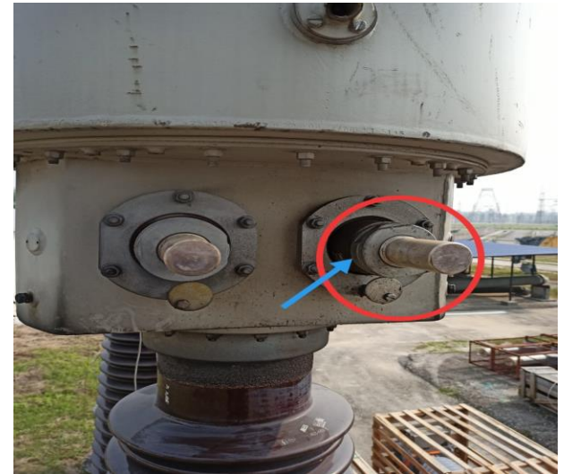
CT oil leakage pics detected by visual inspection
