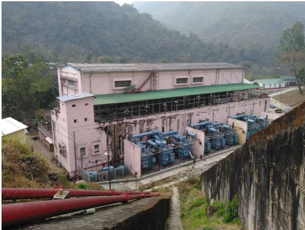
Loktak Hydro Electric Power Plant, NHC
