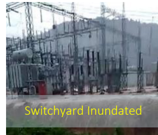
Water through Substation
