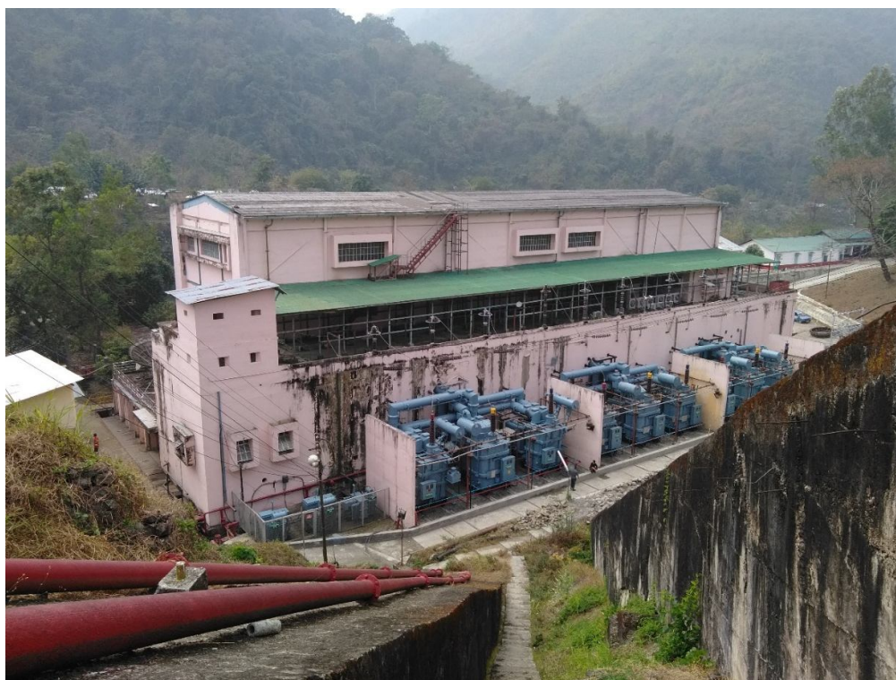
Loktak Hydro Electric Power Plant, NHC
